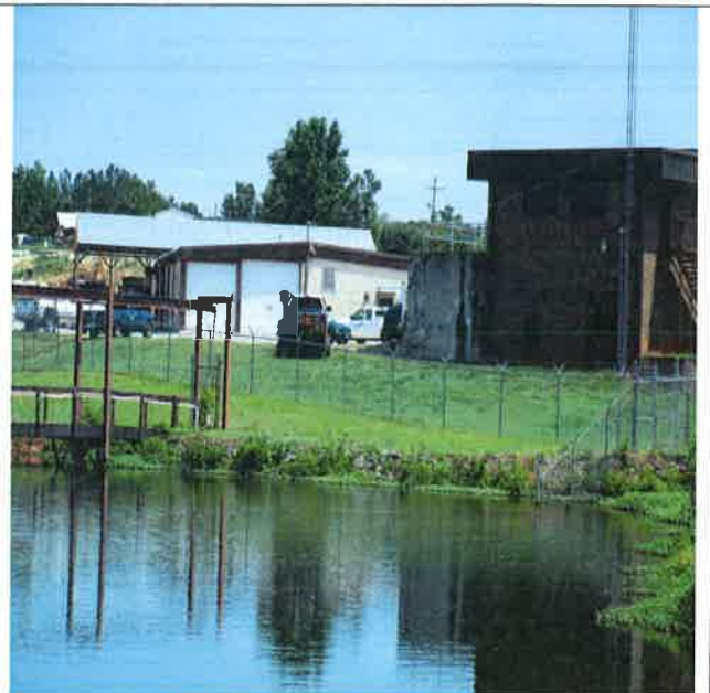
Side banks well maintained
