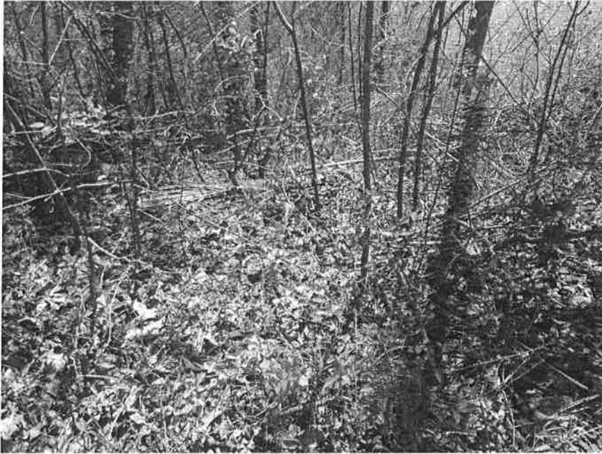
Extreme vegetation on the down slope needs to be removed.
