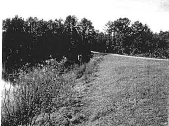
D-0209 Inspection Pictures 12/17/2014
